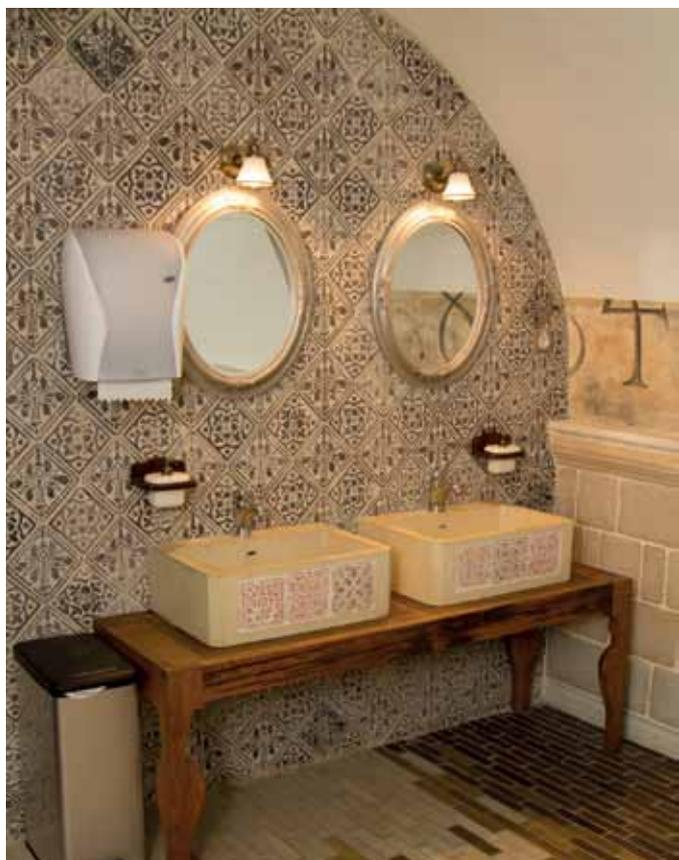
**RIGHT.** To obtain a satin effect finish for the tiles, the final treatment was a mixture of MAPELUX OPACA and MAPELUX LUCIDA protective wax.
