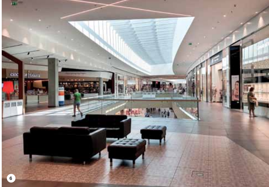
PHOTOS 5 and 6. The two rings of the gallery after completion of the works.
