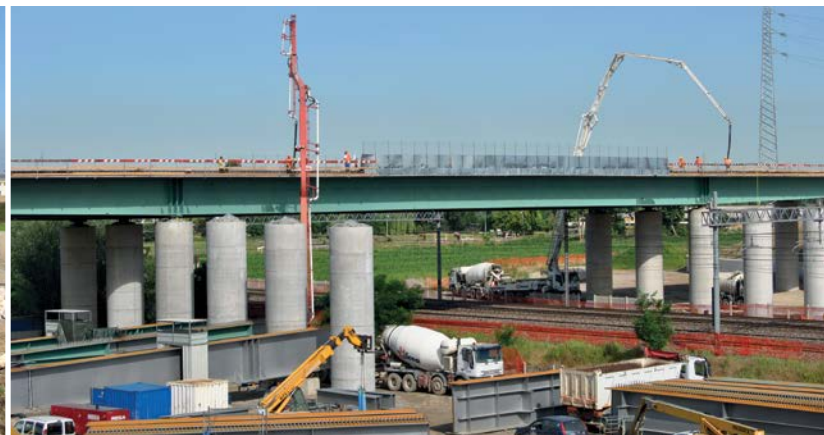
Slab on viaduct
