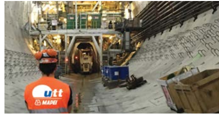
Underground tunneling products
