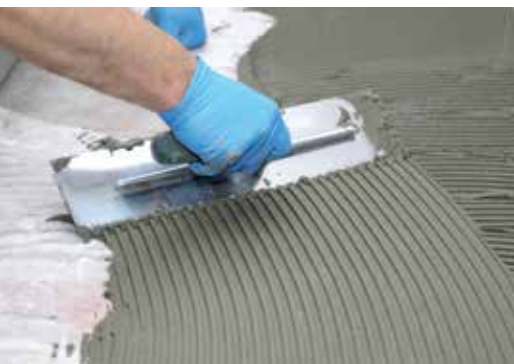
Trowel polymer-modified mortar onto the subfloor.
