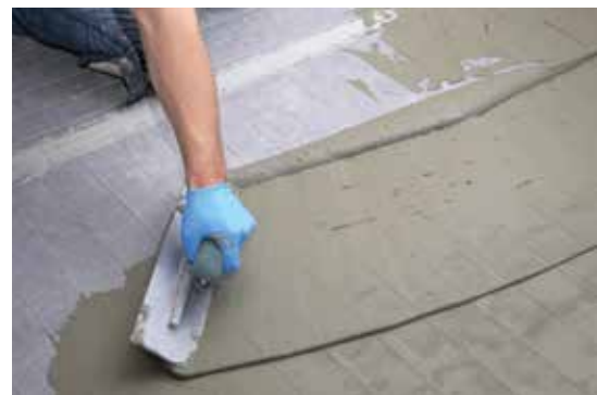
Trowel over with mortar and install tile.
