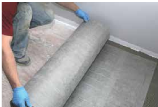
Roll Mapeheat Mat into the fresh mortar.
