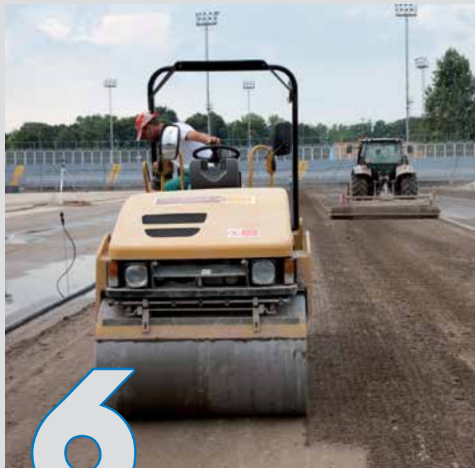
Compacting and curing
