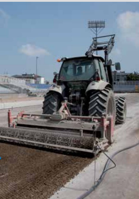
Mixing of Mapesoil 100 with aggregate
