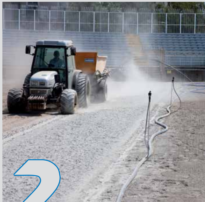
Spreading of Mapesoil 100
