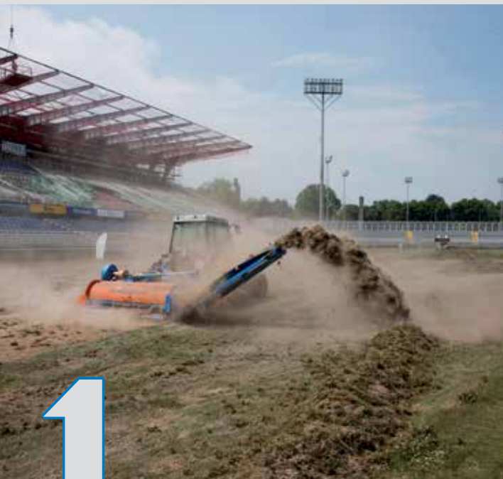
Preparation of soil (topsoil removal)
