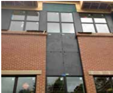
Gauged porcelain tile panels/slab on an exterior facade
