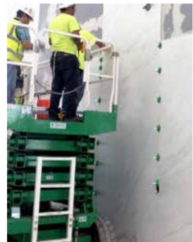
Gauged porcelain tile panels/slab on an interior wall
