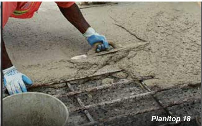
8. **Planitop® 23** two-component, vertical, overhead and horizontal repair mortar can be applied to a depth of 4" (10 cm) in two lifts.
