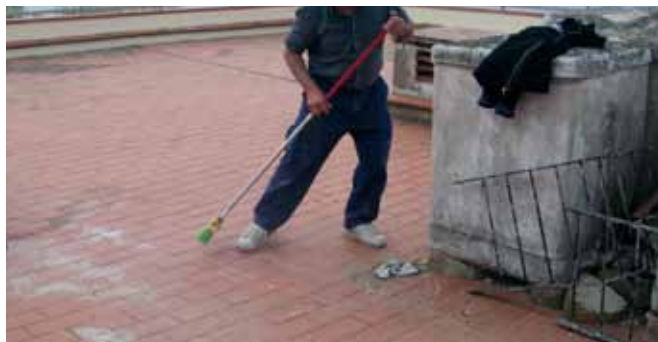
Cleaning a substrate before applying Aquaflex Roof
