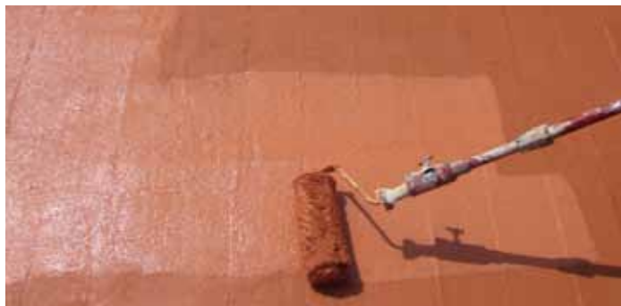
Application of Aquaflex Roof with a long-haired roller
