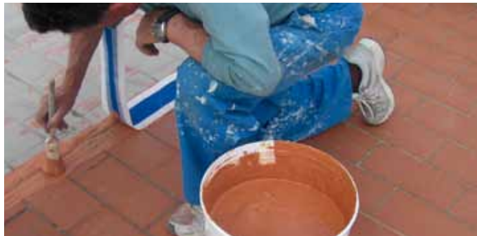
Waterproofing fraction joints with Mapeband fixed with Aquaflex Roof
