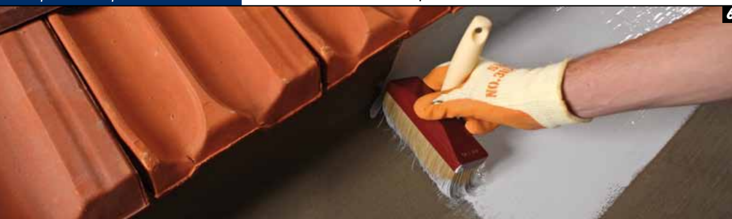
6. Waterproofing of a cement gutter with Mapelastic Smart
