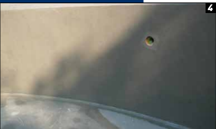
4. Waterproofing of a swimming pool with Mapelastic
