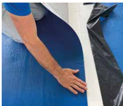
Longitudinal overlaps between rolls.
