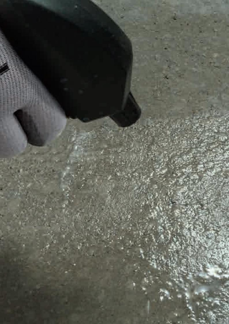
WATER-REPELLENT PRODUCTS FOR THE PROTECTION OF CONCRETE
