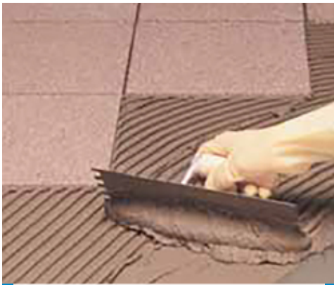
Example of porcelain gres laid on Mapelast using Ultraflex S2 Quick
