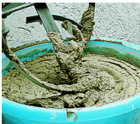
Mixing with a mini cement-mixer
