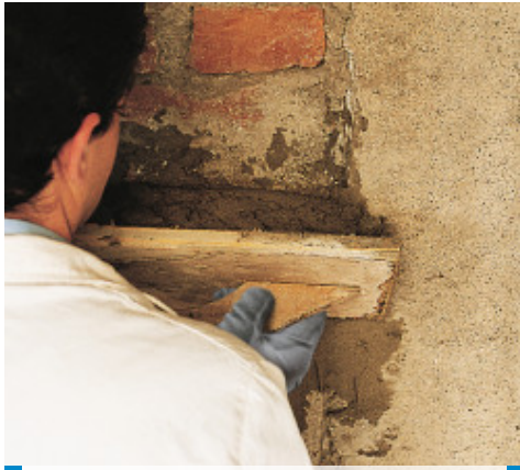
Application of Nivoplan with a float
