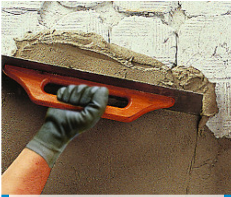
Levelling off the render with a straight-edge
