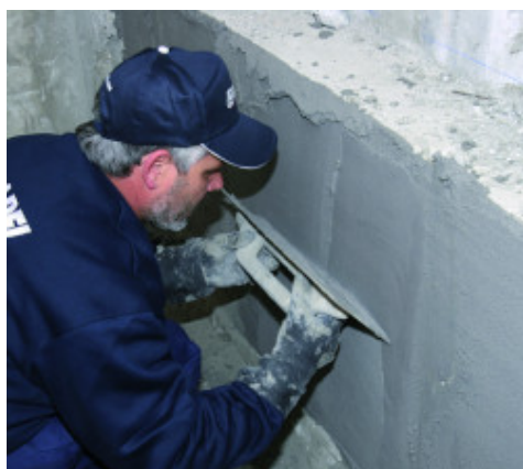
Restoring old brickwork
