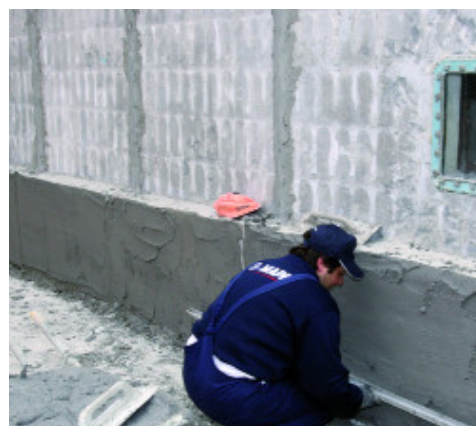
Levelling with a laying-on trowel
