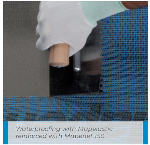
Waterproofing with Mapelastic reinforced with Mapenet 150
