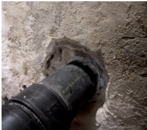
Mapeproof Swell after application
