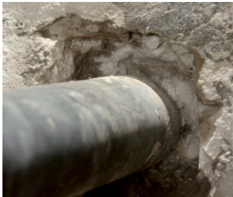
Breaking out the structure around a pipe
