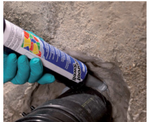
Applying Mapeproof Swell around a pipe
