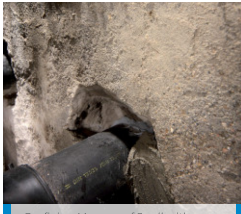
Confining Mapeproof Swell with Mapegrout T40
