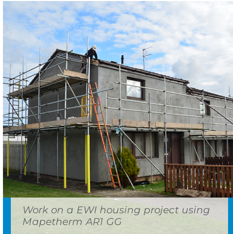
Work on a EWI housing project using Mapetherm ARI GG
