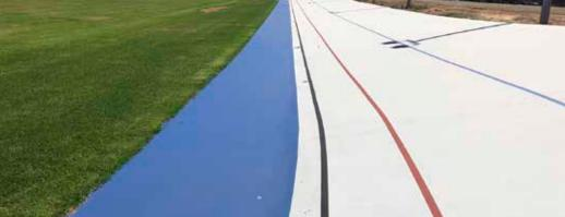
for any period of time, as they can lead to delamination of the acrylic surface. It is recommended to prevent growth of trees either close to or overhanging the velodrome as damage can result from above and/or below the surface.
