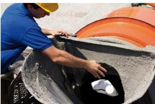
Image 2 – Inserting Re-Con Zero Evo into mixer truck
