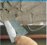
Shrinkage-compensated rapid-setting and hardening fibre-reinforced mortar for repairing concrete.
