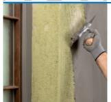
Water-repellent fine-textured cementitious smoothing mortar with a natural finish for concrete and plastic coverings.
