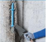
Structural R4-class, rapid-setting, shrinkage-compensated, thixotropic, fibre-reinforced, cementitious mortar, applied in a single layer from 3 to 40 mm thick, for repairing and smoothing concrete.
