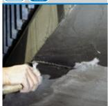
► Medium-strength (40 MPa) thixotropic fibre-reinforced mortar for repairing
