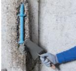
Structural R4-class, rapid-setting, shrinkage-compensated, thixotropic, fibre-reinforced, cementitious mortar, applied in a single layer between 3 and 40 mm thick, for repairing and smoothing concrete
