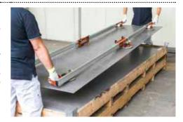
Before handling and moving the tiles, it is recommended to clean the surface of the tile and the suction cups with a damp sponge to get a better grip.
