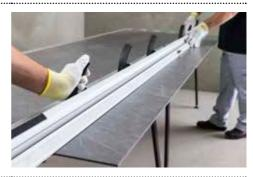
Make a small cut 1 to 2 cm long at each end of the tile from the inside towards the outside.
