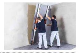
Another essential requirement when installing large format tiles is that the adhesive must guarantee a high level of wetting of the back of the tiles so that gaps are not created, otherwise the soundness and durability of the bond could be affected.
