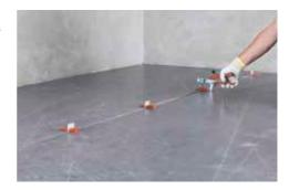
To make this operation easier, a special positioning tool may be used to correct the width of the grout line between adjacent tiles and bring the tiles to the position required.
