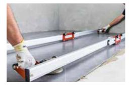
To ensure the tile is completely bonded and that all the air has come out, go over the surface of the tile with a vibro-plate or tap the surface by hand with a special anti-bounce float made from rubber.
