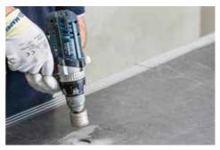
To make rectangular holes in a tile, start by making a round hole at each corner of the rectangle. Then make straight cuts between each hole with a disk cutter with a diamond disk. This will prevent excessive stresses being generated at the corners of the rectangle which could then form a crack in the tile itself.
