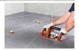
We suggest tapping the tile from the centre working towards the edges in the same direction as the ribs of adhesive, that is, parallel to the short side, to ensure all the air under the tile is forced out.
