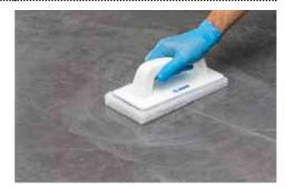
Unlike cementitious grouts, the cleaning of floor and wall tiles grouted with epoxy mortar must be carried out while the grout is still fresh, with a higher amount of water if necessary, in order to completely remove all epoxy resin residuals.
