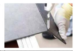
If the edges of the tile are sharp or uneven after it has been broken, clean and smooth the edges with a diamond pad or an abrasive disk.
