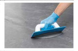
Clean the grout by using a small amount of water and an abrasive pad (such as Scotch-Brite®) followed by a firm cellulose sponge, taking care not to remove the grout.
