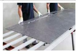
If there is reinforcement mesh in the tile this can be cut and trimmed with a cutter.
