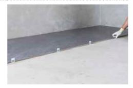
It is important to place the spacers in position before installing the tile and that the spacers are embedded in the adhesive.
