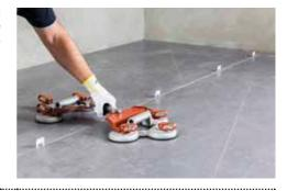
The grout lines may be filled with a cementitious grout, such as **Keracolor FF**, **Keracolor GG** or **Ultracolor Plus** or with an epoxy grout such as **Kerapoxy** or **Kerapoxy Design**.
