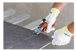
The tile is then broken in two by simply bending it until the two pieces come apart.
