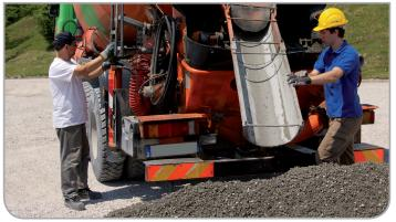
After mixing for a few minutes with **RE-CON** ZERØ or **RE-CON** ZERØ **EVO**, concrete is transformed into granular material which may be discharged on the ground and, once cured, used as aggregate in concrete. **RE-CON** ZERØ or **RE-CON** ZERØ **EVO** work with all types of concrete.
