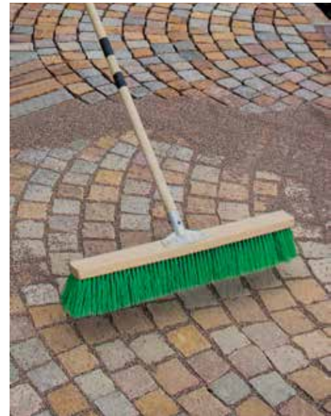
Fill the grout lines with 2/4 mm medium stone chippings
