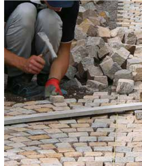
Install the stone blocks on a bed of 4-8 mm coarse stone chippings
