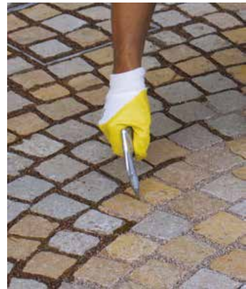
Fill the grout lines with Mapestone Joint resin
