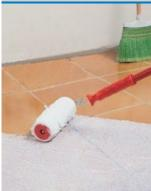
➤ Two-component, solvent free primer to ensure perfect bonding with smoothing and levelling compounds and cementitious mortars on non-absorbent and difficult substrates - very low VOC
