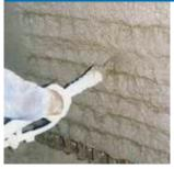
One-component shrinkage-compensated sulphate-resistant thixotropic fibre-reinforced mortar applied with a rendering machine, particularly suitable for repairing concrete structures.
