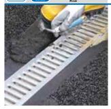
Rapid-setting and hardening shrinkage-compensated thixotropic mortar for repairing concrete and anchoring drains, manholes and urban features and highway coating materials.
