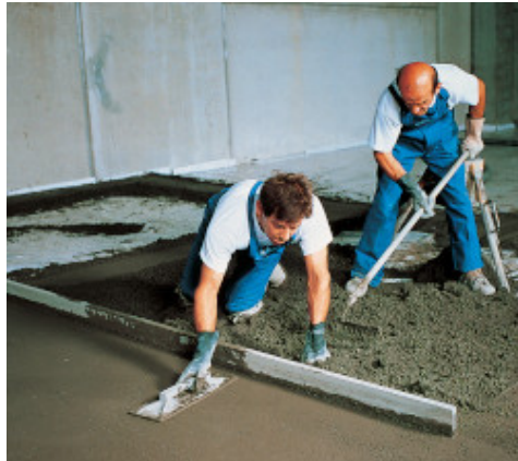
Tamping the Mapecem screed
