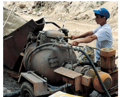
Mixing Mapecem with an automatic pumping unit
