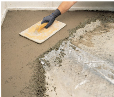
Covering pipes with Mapecem and reinforcement netting
