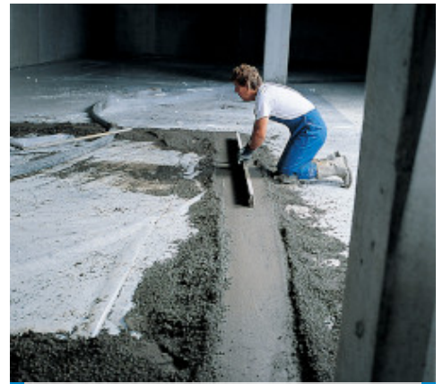
Preparing a levelling strip
