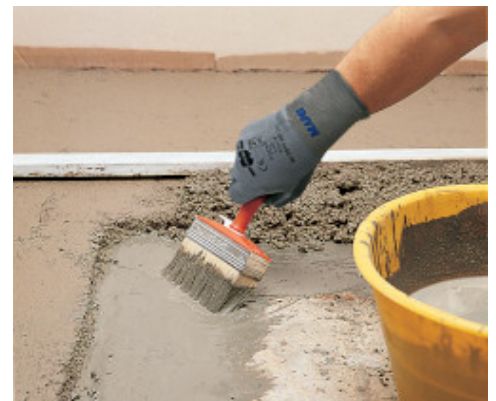
Spreading the anchoring slurry for bonded Mapecem screeds
