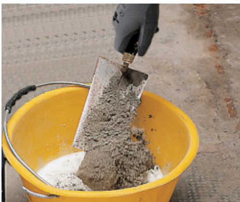
Mixing Mapecem with Planicrete SP to make a bonding slurry
