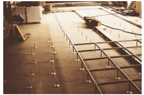
Slab levelled with Ultraplan ready for fixing a floating floor
