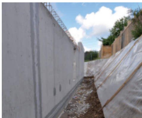
Sealing structural joints in retaining walls
