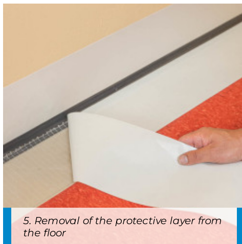
2. Removal of part of the protective layer of the dimensions of the cove former
