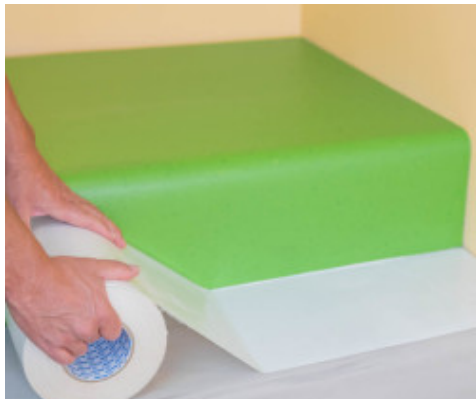
1. Placement of Mapecontact Plus on the tread and then on the riser
