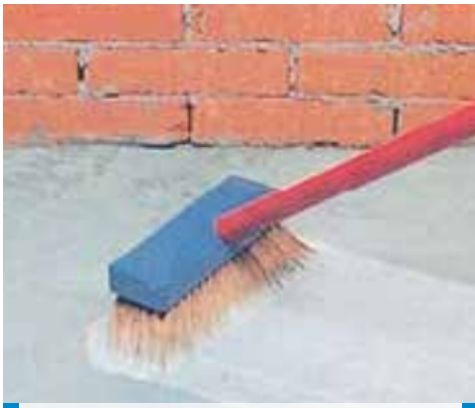
Applying cement slurry modified with Planicrete SP
