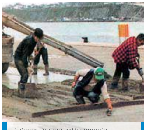
Exterior flooring with concrete admixed with Planicrete SP.
