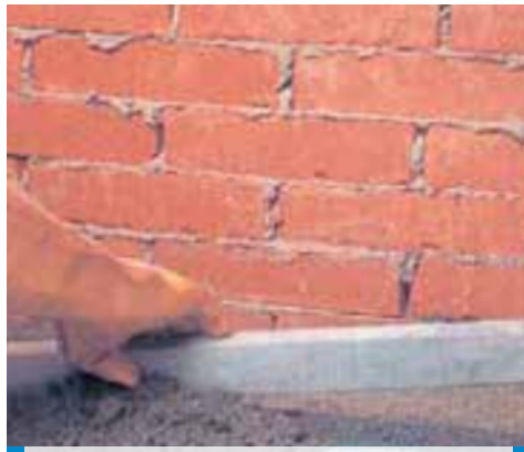
Applying cement screed modified with Planicrete SP
