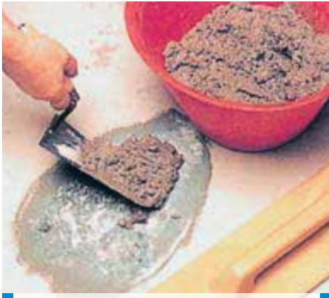
Floor patching: application of mortar
