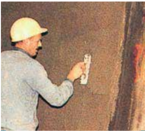
Cement plaster with Planicrete SP.
