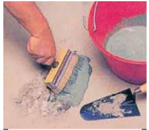
Floor patching: application of slurry
