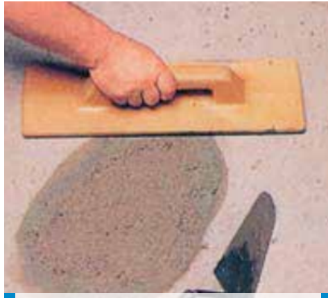
Floor patching: final smoothing
