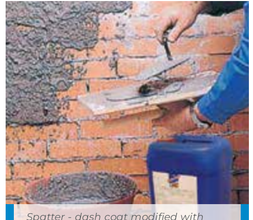
Spatter - dash coat modified with Planicrete SP
