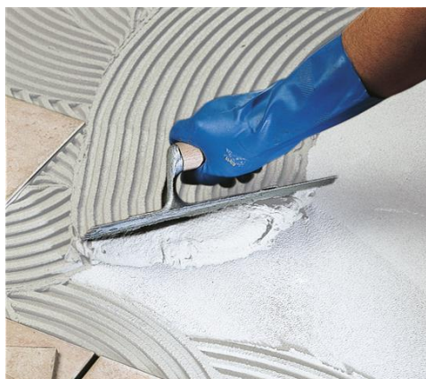
Installation of single-fired tile on floor
