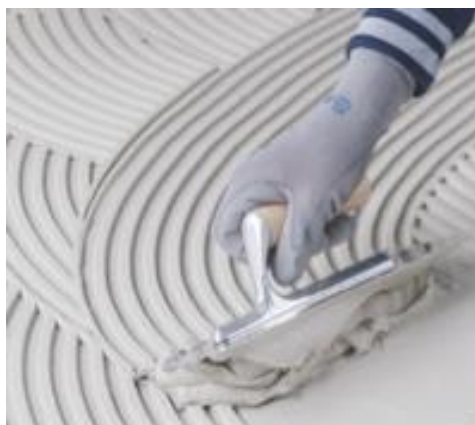
Spreading Adesilex P9
