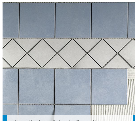
Installation of single-fired tile on gypsum board wall
