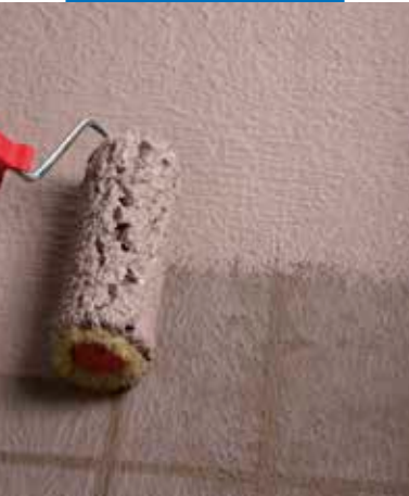
Waterproofing of details by roller
