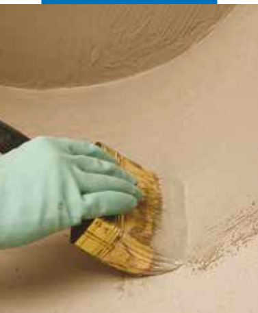
Waterproofing of details by brush
