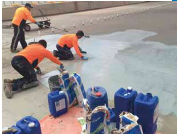
Installing Mapelastic Smart in the 50 metre pool at the Adelaide Aquatic Centre
