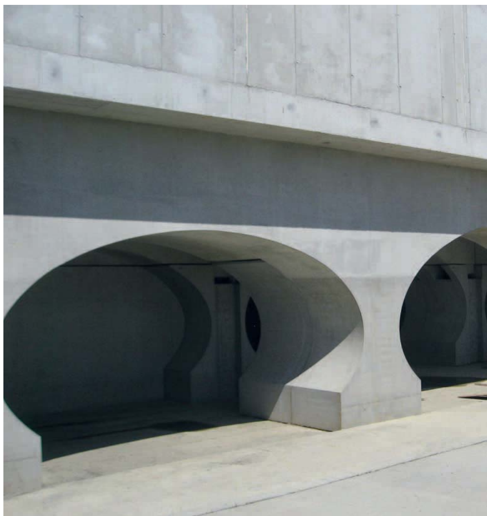
Tunnel in offener Bauweise in Hankenfeld
