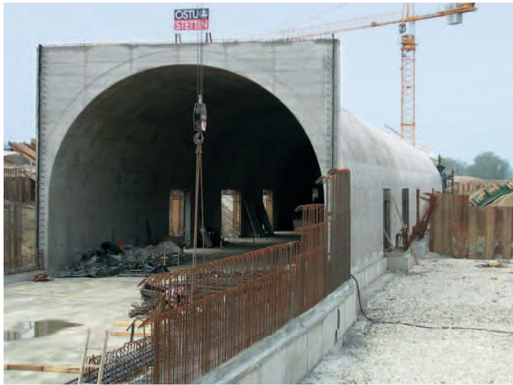
Tunnel in offener Bauweise in Hankenfeld
