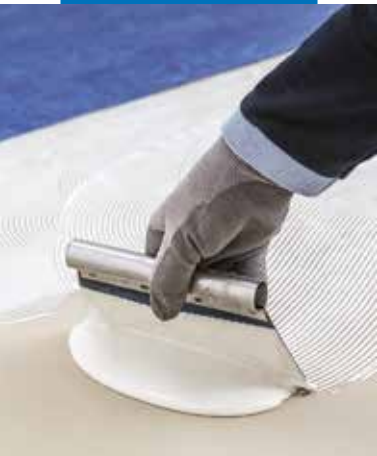
Use of Ultrabond Eco VS30 for laying linoleum
