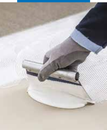
Use of Ultrabond Eco VS30 for laying carpet
