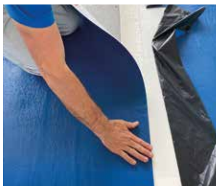
Longitudinal overlaps between rolls.
