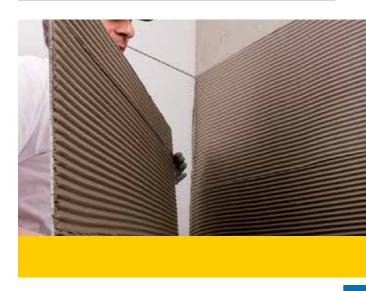
One-component, high-performance, highly deformable, lightweight cementitious adhesive with extended open time for ceramic tiles, natural stone and thin porcelain tiles.
