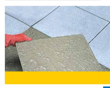
High-performance, self-buttering, rapid-setting grey cementitious adhesive for ceramic tiles and natural stone.
