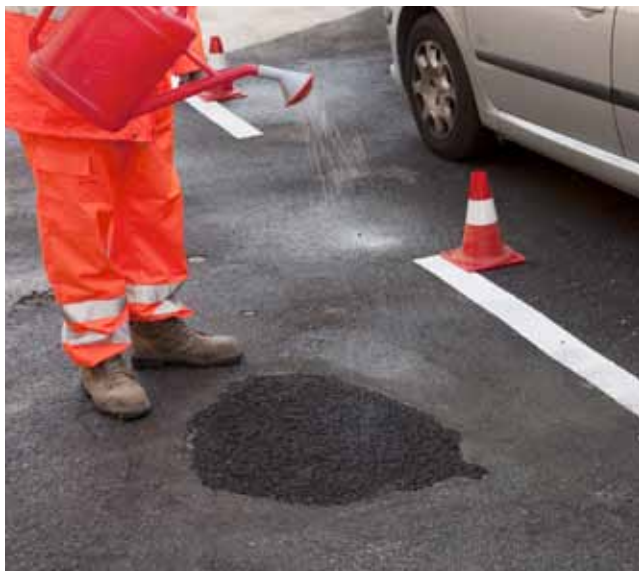
3. Wetting the surface of Mape-Asphalt Repair 0/8
