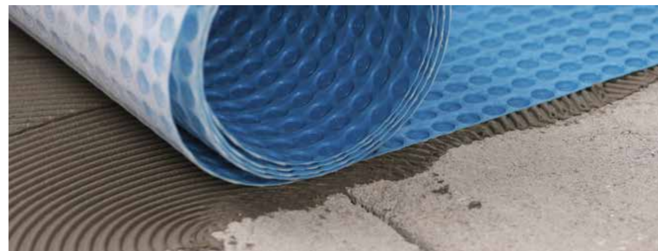
Laying Mapeguard UM 35 on a cementitious screed with control joints.
