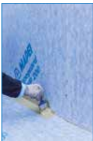
Application of Mapeguard WP Adhesive to bond Mapeguard ST
