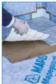
Installation of glass mosaic on Mapeguard WP 200
