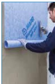
Application of Mapeguard WP 200
