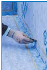
Application of Mapeguard ST
