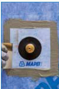
Application of Mapeguard PC
