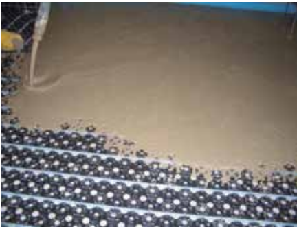
Applying Novoplan Maxi to create a thin heated floor
