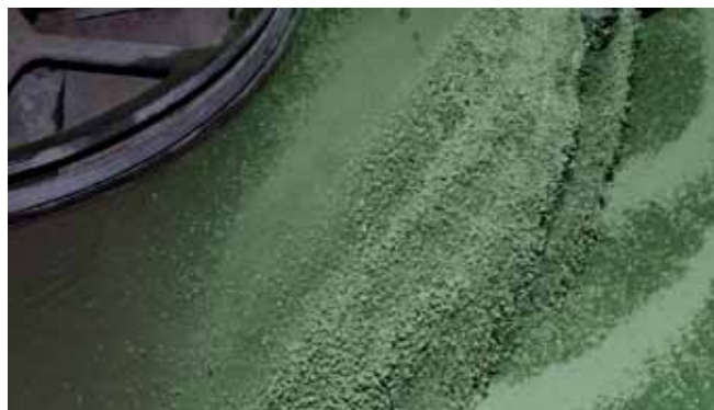
Manual application of Mapetop N AR6
