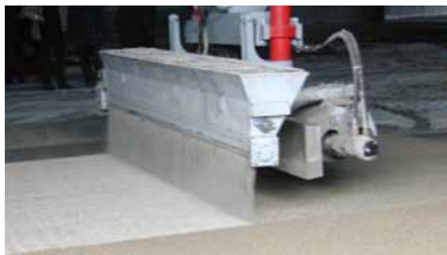
Mechanical application of Mapetop N AR6
