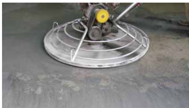
Levelling the surface using a vibro-compacting machine
