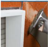
Water-repellent coarse-textured cementitious smoothing mortar with a natural finish for concrete and plastic coverings.
