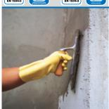
One-component normal-setting cementitious mortar for smoothing concrete and cementitious render.
