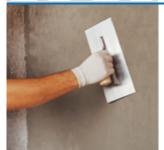
Water-repellent fine-textured cementitious smoothing mortar with a natural finish for render and concrete.
