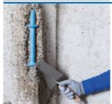
Structural R4-class, rapid-setting, shrinkage-compensated, thixotropic, fibrereinforced, cementitious mortar, applied in a single layer from 3 to 40 mm thick, for repairing and smoothing concrete.
