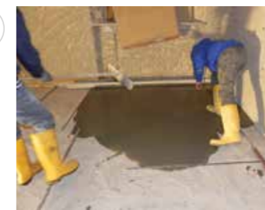
Level off the surface
