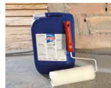
Consolidate the surface with Primer 3296
