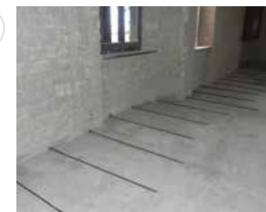
Anchor around the edges with steel bars
