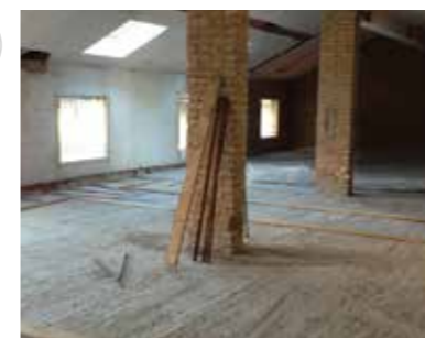
Roughen the substrate
