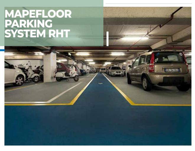
Multi-layered, seamless epoxy system for pedestrian areas and surfaces with vehicle access exposed to intense traffic. The system complies with the Guidelines of the German Committee on Reinforced Concrete OS 8 and the concrete surface protection systems according to EN 1504-2; thickness 3 to 3.5 mm.
