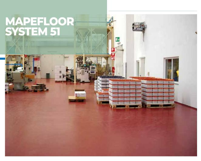
Multi-layered vapour-permeable epoxy system in water dispersion with a matt non-slip finish for industrial floors; average thickness 3 mm.
