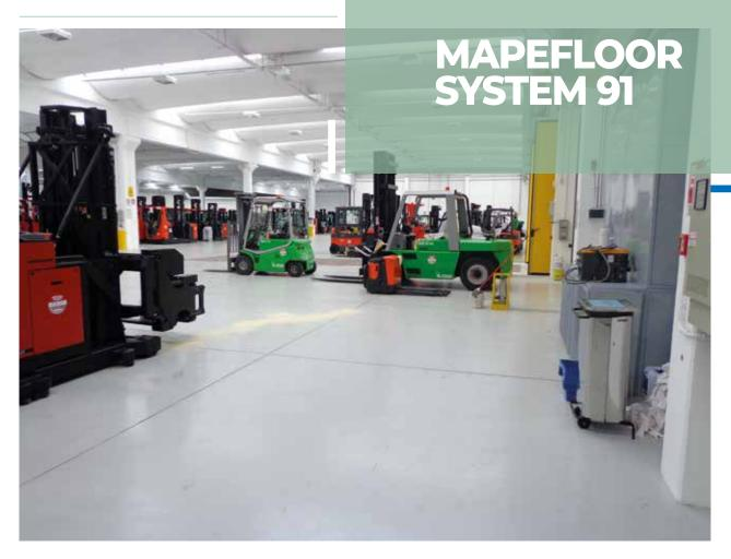
Trowelled epoxy mortar system for industrial floors, ideal for renovating old floors; thickness 6 to 15 mm.
