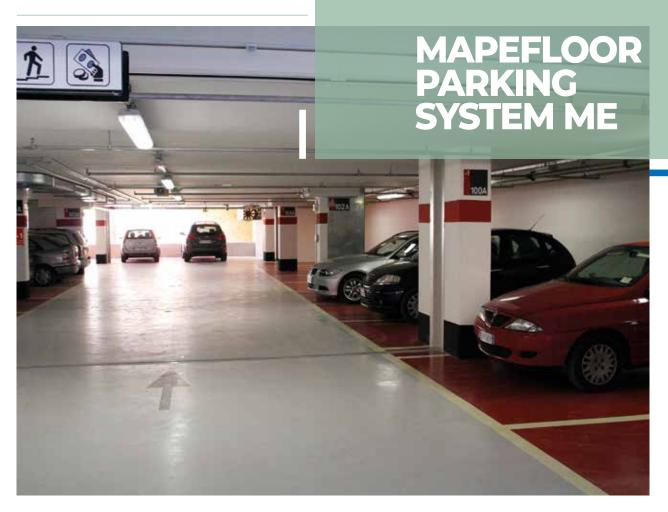
Multi-layered, seamless polyurethane system with high dynamic crack-bridging capacity for pedestrian surfaces and areas with vehicle access exposed to intense traffic also outdoor. The system complies with the Guideline of the German Committee on Reinforced Concrete OS 11b and the concrete surface protection systems according to EN 1504-2; thickness 4 to 4.5 mm.
