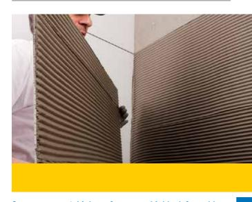
One-component, high-performance, highly deformable, lightweight cementitious adhesive with extended open time for ceramic tiles, natural stone and thin porcelain tiles.
