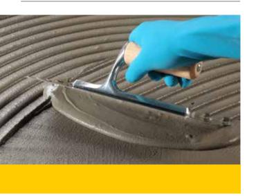
Easy-to-apply, high-performance, deformable cementitious adhesive with extended open time and high wetting capacity for ceramic tiles and natural stone.
