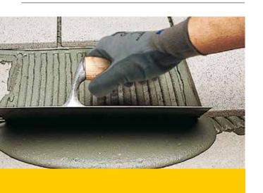
Two-component, high-performance, deformable, rapidsetting and hydrating cementitious adhesive for ceramic tiles and natural stone.
