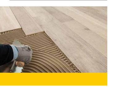
One-component, high-performance, non-slip, lightweight cementitious adhesive with moderate deformability and extended open time for ceramic tiles, natural stone and slim porcelain tiles.
