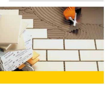
Two-component, high-performance, highly-deformable, rapid-setting and hydrating, non-slip cementitious adhesive with extended open time for ceramic tiles and natural stone.
