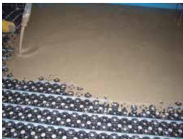
Applying **Novoplan Maxi** to create a thin heated floor
