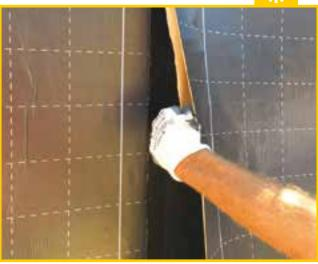
Membrane suitable for application at high temperatures up to +45°C
