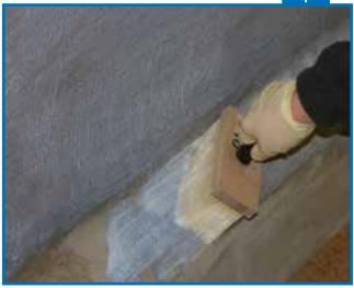
One-component primer for membranes applied at low temperatures
