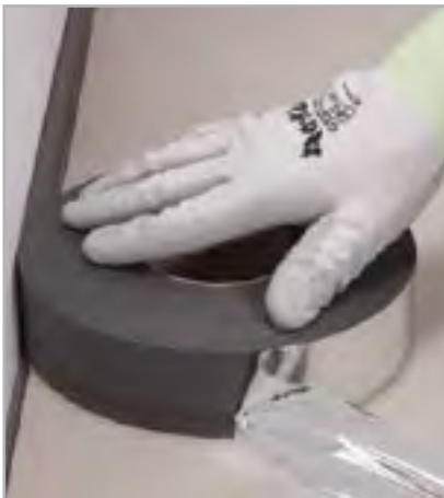
Fig. 5.2 - Apply MAPESONIC STRIP around the perimeter
