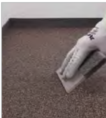
Fig. 5.5 - Massage the surface of MAPESONIC CR
