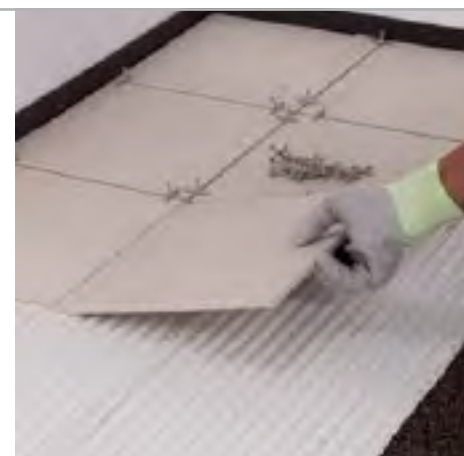
Fig. 5.6 - Spread the adhesive to bond ceramic tiles
