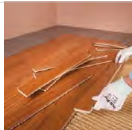
Fig. 5.7 - Spread the adhesive to bond parquet
