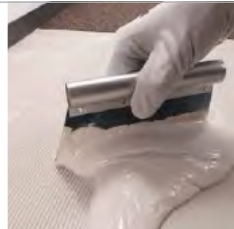
Fig. 5.3 - Spread on the adhesive to bond MAPESONIC CR
