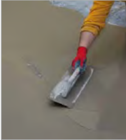
Fig. 5.1 - Levelling of the substrate
