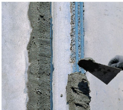
Application with trowel
