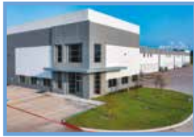
New facilities in the USA and Portugal USA - PORTUGAL
